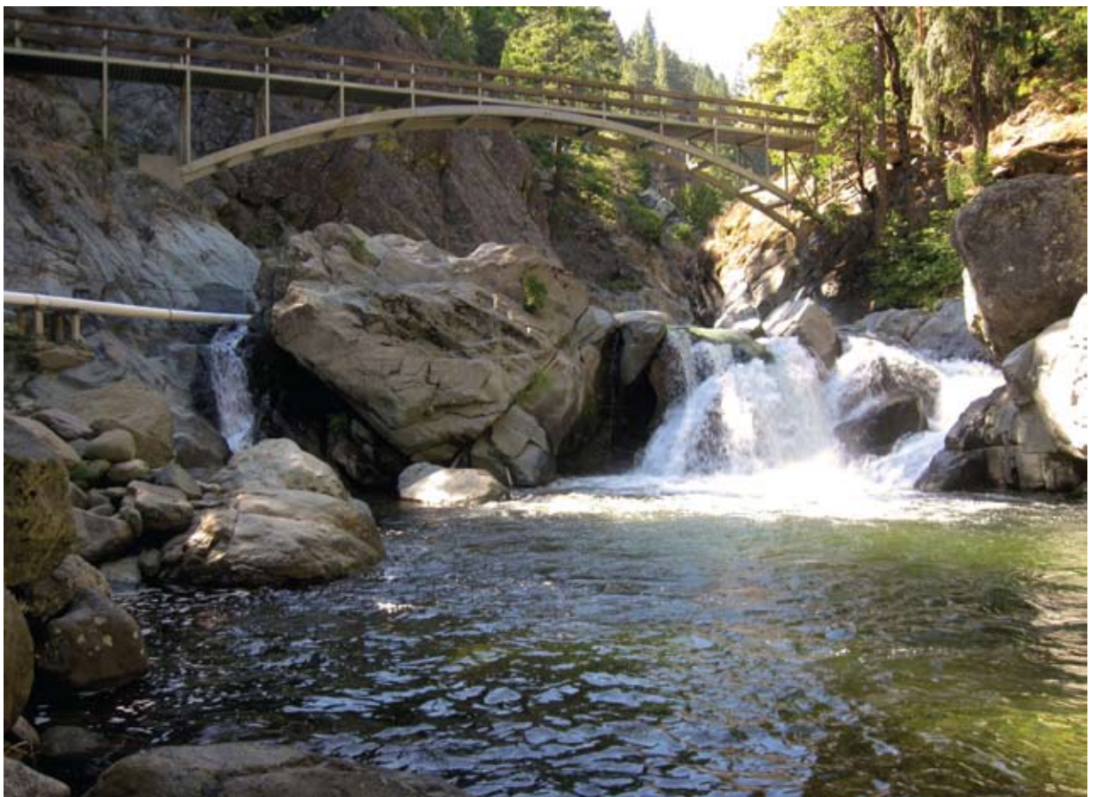
North Yuba near Pacific Crest Trail 4
