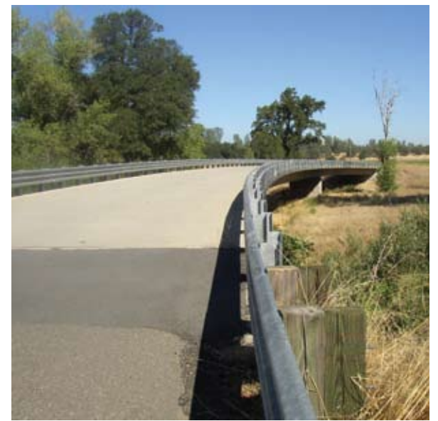
Parkville bridge over Bear Creek
