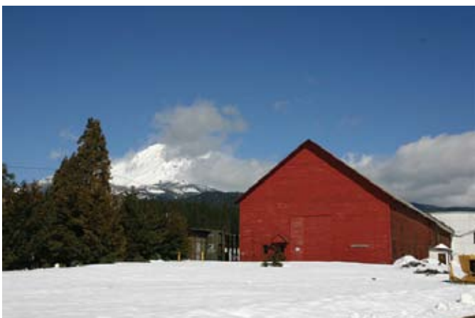
Storage barn at McCloud Railroad 3
