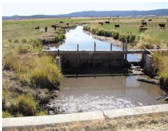
Irrigation diversion dam on Pit River tributary (Willow Cr)
