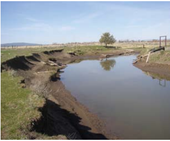
Degraded channel and riparian habitat on Pit River near Bieber
