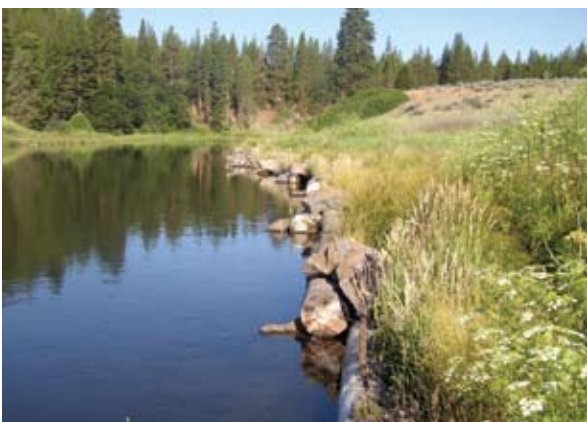
DFG bank stabilization project (erosion from muskrats)
