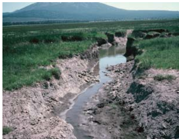
Burney Creek channel erosion
