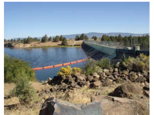
PG&E Pit 1 diversion (from above)
