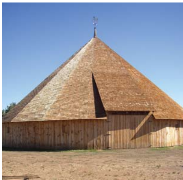
'The round barn' recently restored in Fall River Mills
