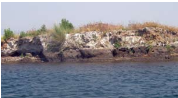
Bank erosion from muskrat borrows
