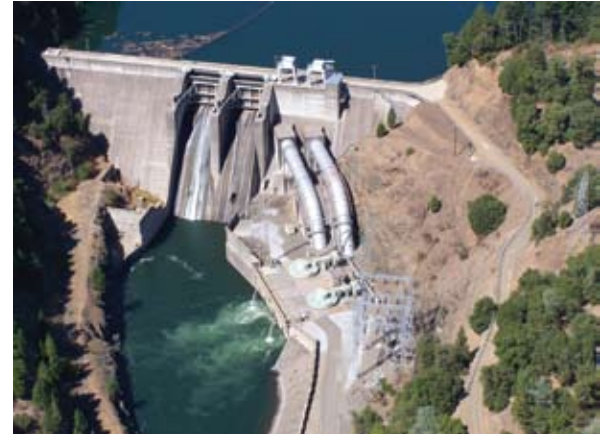
PG&E Pit 6 Dam
