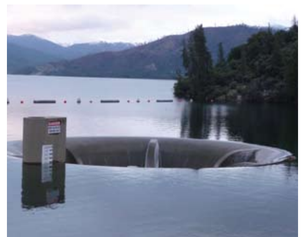
Whiskeytown Reservoir and 'Glory Hole' spillway
