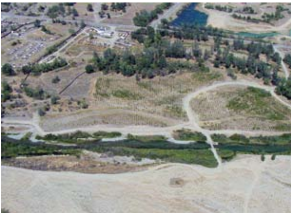
Restoration Grove, site of Clear Creek channel and riparian improvement project
