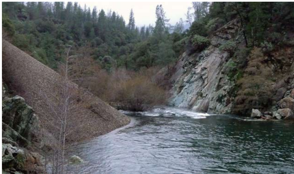
Stockpile for stream gravel augmentation
