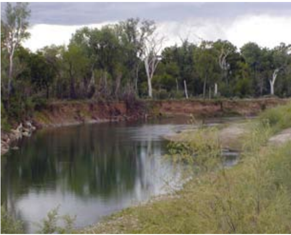
Channel erosion on Lower Cottonwood Creek
