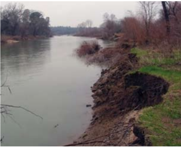
Channel erosion on Lower Cottonwood Creek
