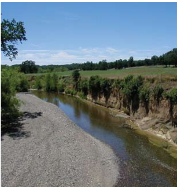
Red Bank Creek erosion
